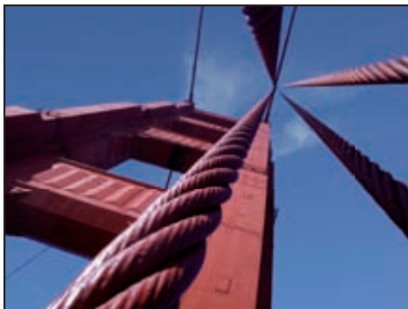
32 km of the Golden Gate bridge's cables are protected by NOXYDE®
