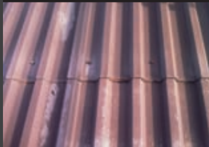
Old Plastisol® roof BEFORE
