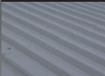
Plastisol® roof AFTER
