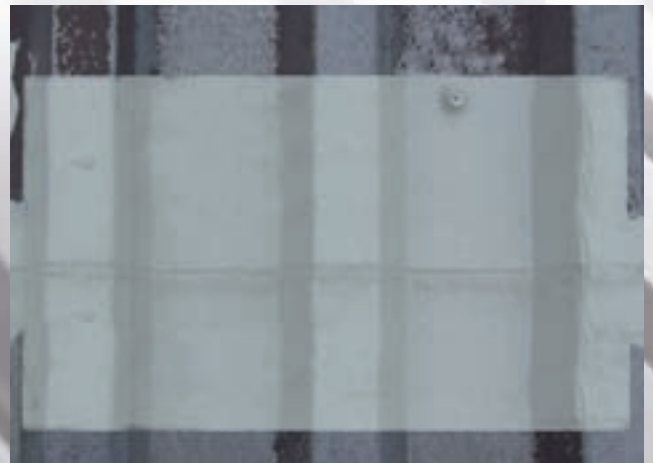
Edge lap after treatment with Noxyde®/Elastofill®
